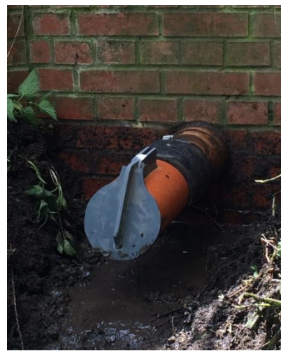
Newly installed flap valves in Crown Street
