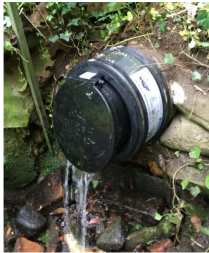
Newly installed flap valves in Crown Street
