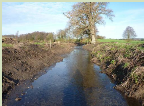
These photos show a couple of examples of where bank and bed material has been removed from the river – the sort of damage we are keen to avoid.
