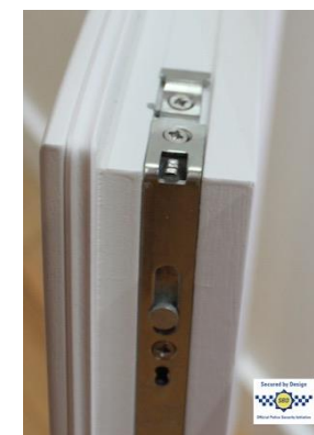
Multi-point locking mechanism (Source: Sashed)
